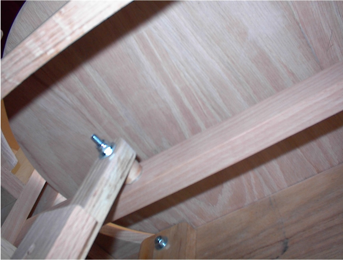
Fig. 37 Upper Link Connection
