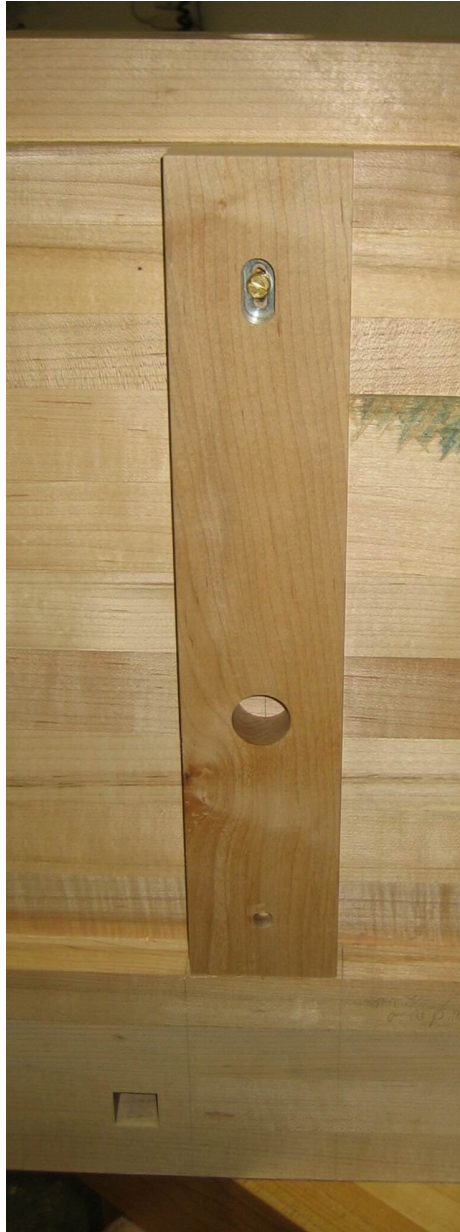
Figure 54: View of underside filler strip
