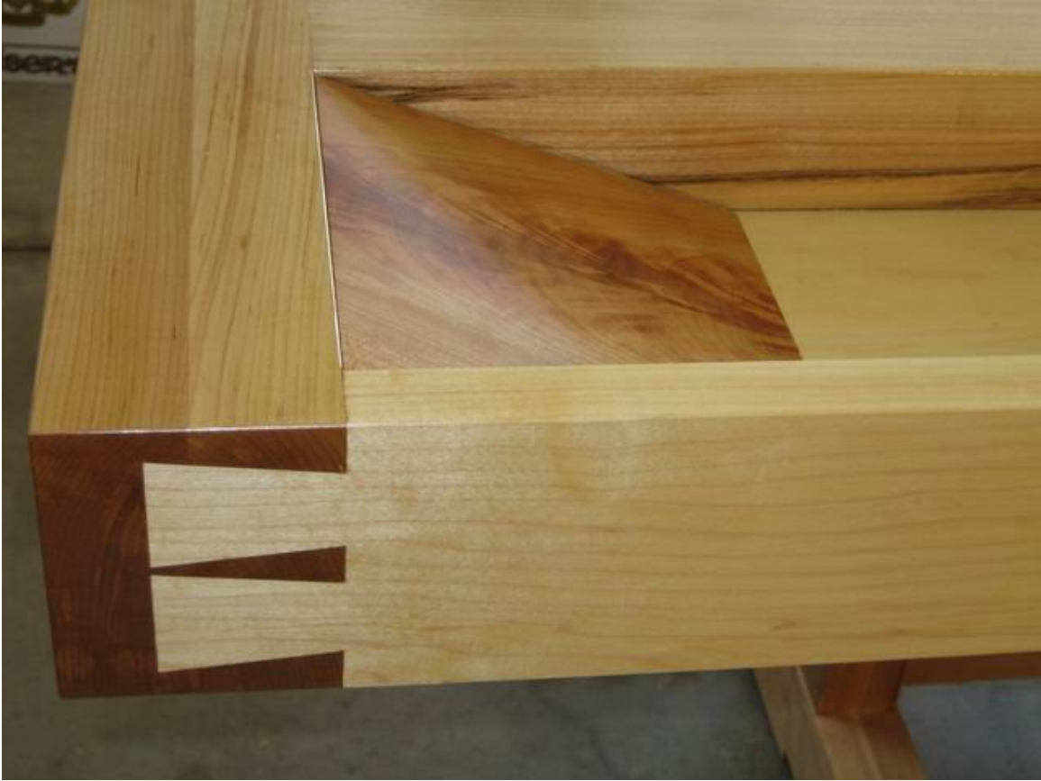
Figure 10: Tool tray dovetails
