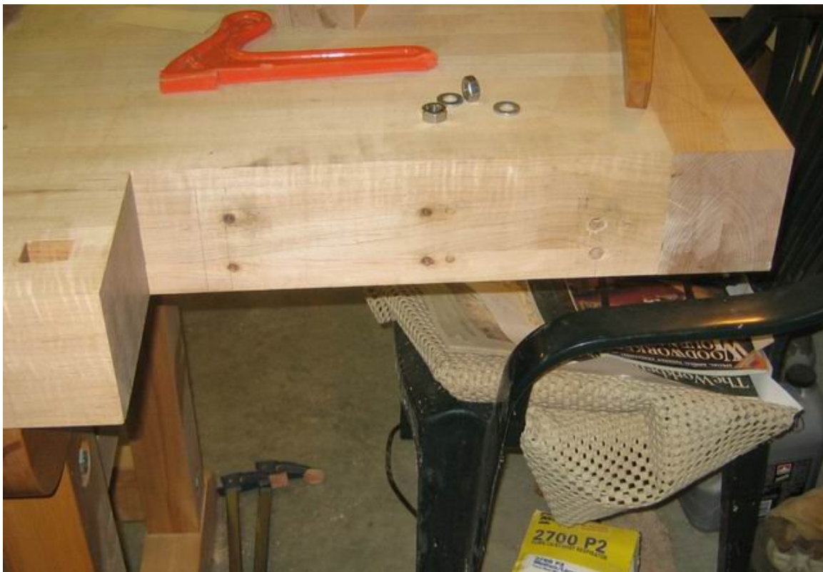
Figure 79: Screw and bolt holes - note the dirty marks on the wood are because I screwed the plate into the wrong location the first time and had to plug the holes with dowels and drill new holes
